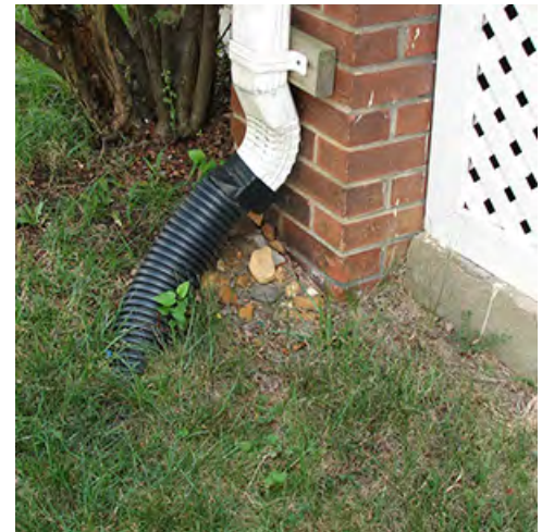
Figure 17. Extending downspouts at their base is one of the basic steps to reduce dampness in basements, crawl spaces and around foundations. Extensions should be buried, if possible, for aesthetics, ease of lawn care, and to avoid creating a tripping hazard. Photo: NPS files.
