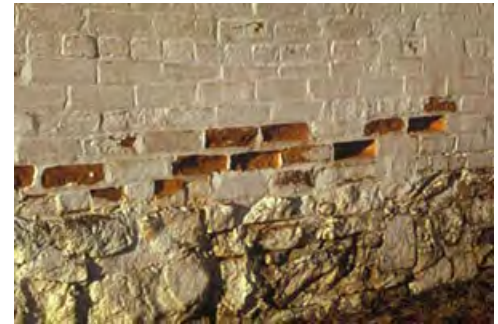
Figure 10. Repointing of masonry should usually be approached as repair rather than maintenance work in part because of the need for a skilled mason familiar with historic mortar. In this case, a moisture condition was not corrected and the use of a waterproof coating and off-the-shelf Portland cement mortar trapped water and resulted in further damage to these 19th century bricks. Photo: NPS files
