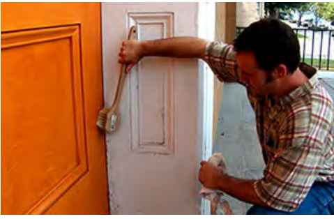
Figure 9. To help extend a repainting cycle, dirt and spider webs should be removed before permanent staining occurs. In this case, a natural bristle brush and a soft damp cloth are being used to remove insect debris and refresh the surface appearance.
