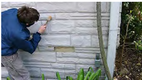
Figure 6. Stucco applied to an exterior wall or foundation was intended to function as a watertight surface. Unless maintained, rainwater will penetrate open joints and cracks that may occur over time. A small section of stucco indicates some damage has occurred and a wooden mallet is being used to tap the surface to determine whether the immediate stucco has lost adhesion. Photo: Bryan Blundell.
