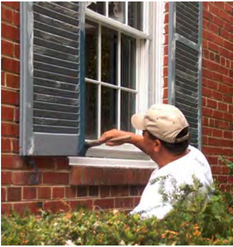
Figure 12. Good surface preparation is essential for long lasting paint. Scraping loose paint, filling nail holes and cracks, sanding, and wiping with a damp cloth prior to repainting are all important steps whether touching up small areas or repainting an entire feature. Always use a manufacturer's best quality paint. Windows and shutters may need repainting every five to seven years, depending on exposure and climate.
