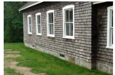
UC-7 Pitch grade away from foundation
