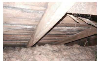
MH-9 Broken roof sheathing
