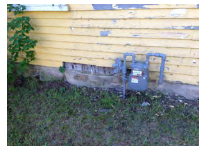
KH-10 Missing clapboard
