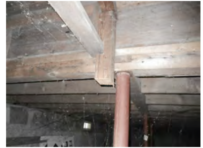
UC-16 Center beam supported by columns
