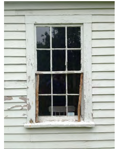
DS-10 Existing 6/6 wood double-hung window
