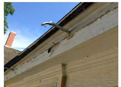
KH-14 Existing gutter hangers
