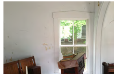
UC-13 Typical interior plaster cracks
