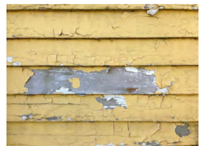
KH-9 Failed exterior paint – typical
