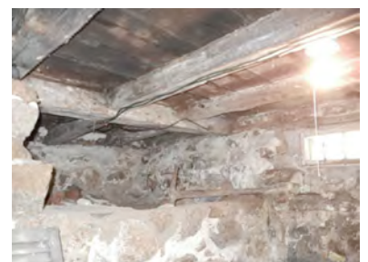
FT-16 First floor framing
