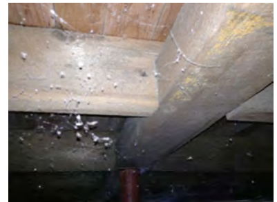
UC-17 Joists notched into beam
