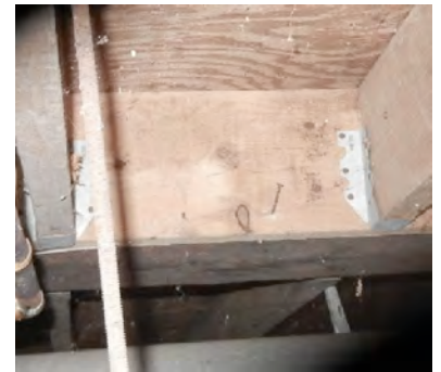
MH-17 Reinforced floor framing
