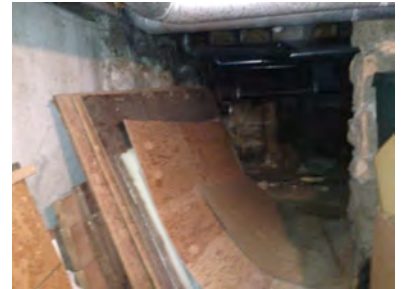
MH-13 Existing basement (conc foundation @ left with fieldstone foundation @right & beyond
