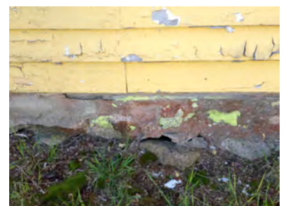
KH-5 Fieldstone foundation needs selective repointing
