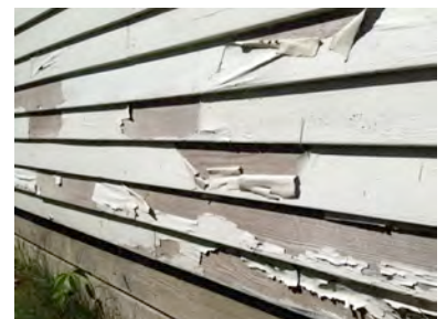
DS-5 Failing paint at east side
