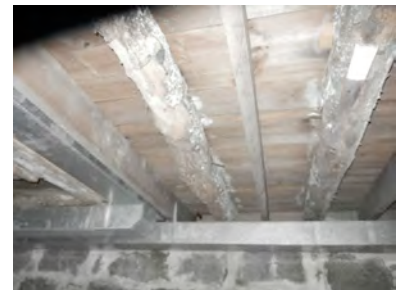
KH-18 Existing framing with reinforcements
