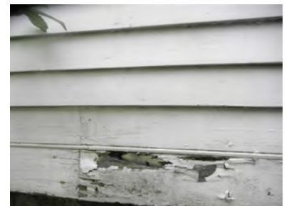
MH-19 Insect damage
