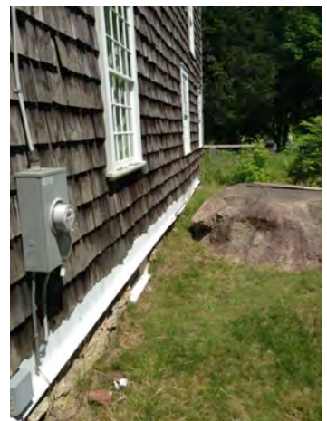
FT-7 Bulging east wall
