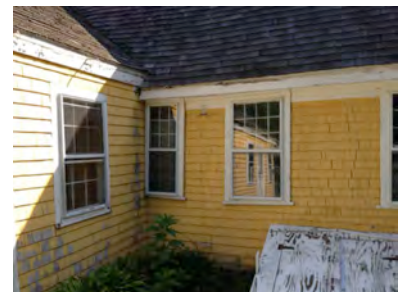
KH-15 Missing downspouts
