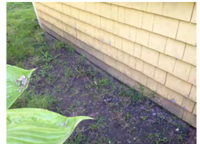
KH-7 Low clearance between grade & siding
