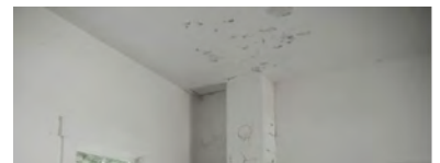
UC-12 Water damage around chimney
