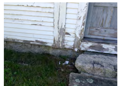
DS-4 Missing masonry joint at storage addition
