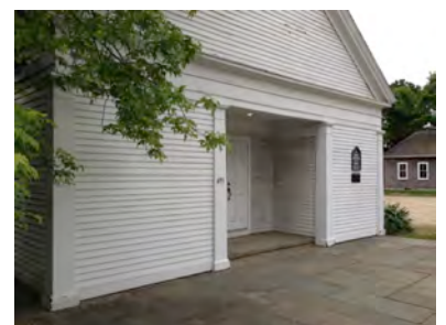
MH-4 Bluestone paving at main entrance
