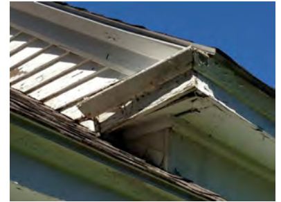
DS-6 Damaged & missing trim at eave
