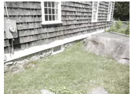
FT-3 East wall bulge behind granite boulder
