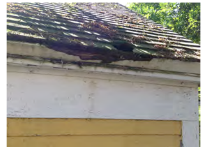
KH-12 Rodent damage at rotten trim
