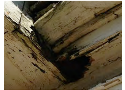
KH-16 Rodent & water damage
